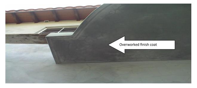
It may be unwise to try to seal all of these cracks and it is generally considered inadvisable where cosmetics are the only reason for doing so. These minor cracks are usually more pronounced after a rain or on a foggy morning as the wall begins to dry out. Often, the repair of this type of crack is more visible than the crack itself. Usually, these cracks can be covered with a good primer and a high-solids latex paint. The owner should decide which direction to go.
